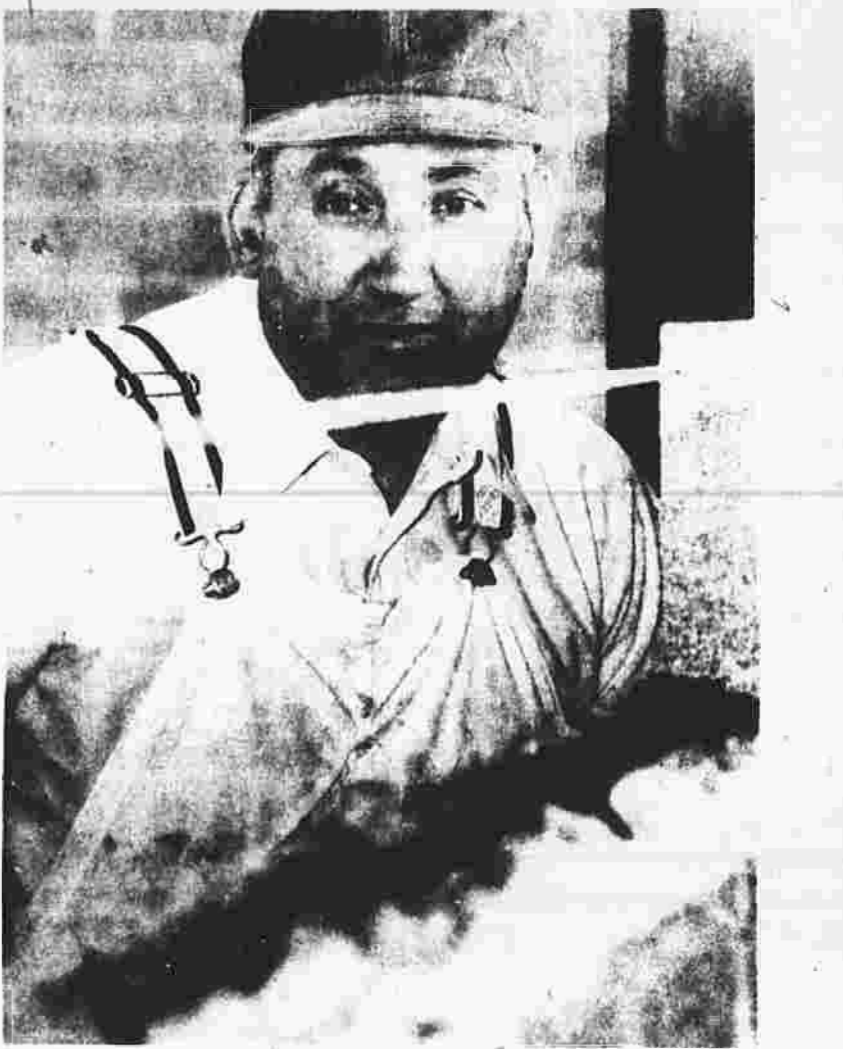
CURT LAASER LAYS MORTAR ... cinderblock corridor wall on second floor
