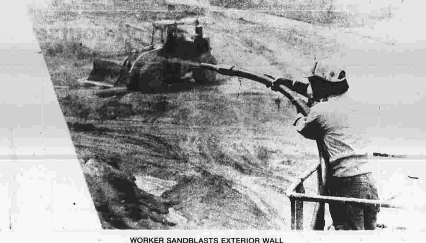
WORKER SANDBLASTS EXTERIOR WALL ... produces uniform finish on concrete
