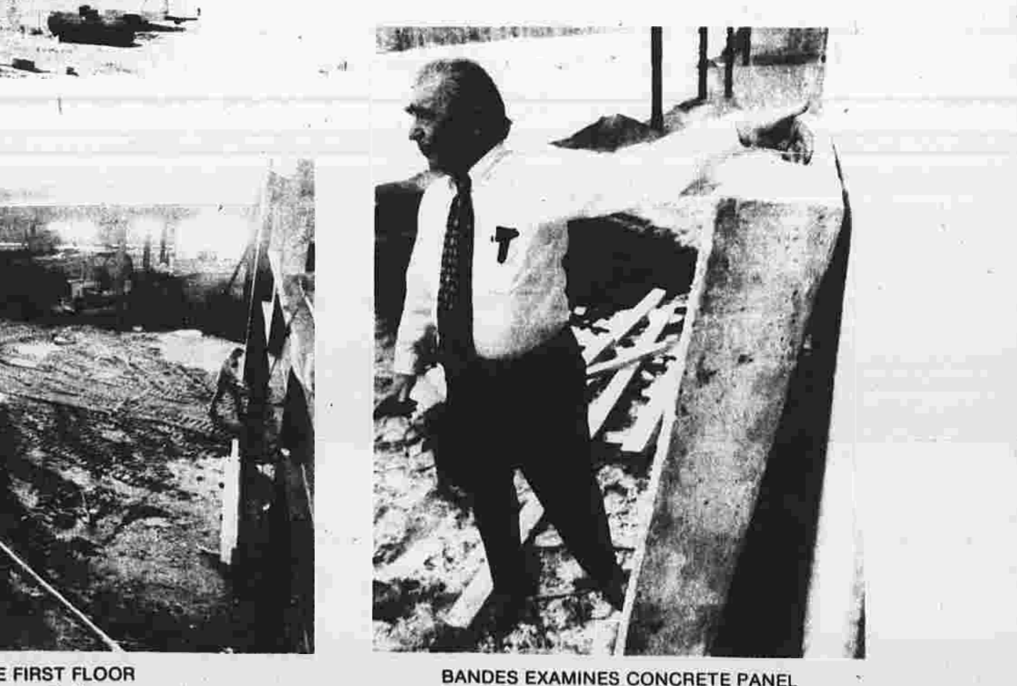
BANDES EXAMINES CONCRETE PANEL ... dean oversees construction progress
